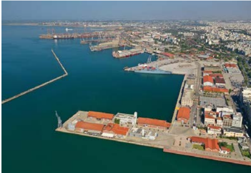
Figure SEQ Figure \* ARABIC 1. View of the first pier of Thessaloniki's port . Source: thpa.gr
