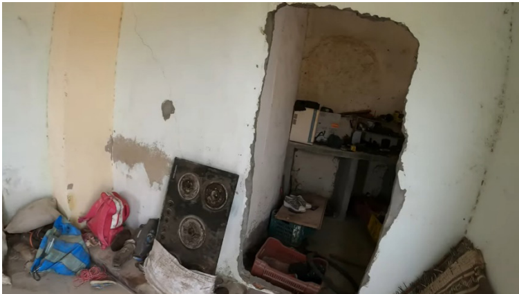
Figure 13. Modification to the building. Source : Hamrouni. (2020).
