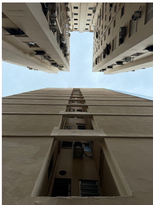
Figure 2. Service Area ventilation shaft and indent in Rio de Janeiro. Source: Photo by the author (2024).
