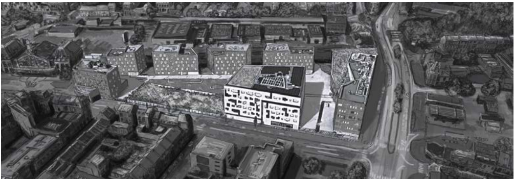
Figure 1: View of the IUT de Lille's building ©Margaux D'Hont
